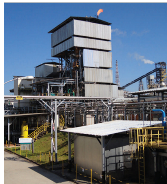
Petrobras' 200 kg/hr (30 bpd) Demonstration FCC
